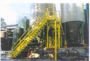
The FRP walkways are built by assembling fiberglass and polyester resin pultruded profiles and gratings; they assure several advantages compared to the normal metal ones:
